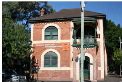
St John's Parish Hall, Glebe
